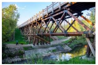
The Mill Creek Ravine is both a recreation destination and commuter link into downtown Edmonton. Working with the City, ISL replaced two pedestrian bridges and restored three historic railway-turned-pedestrian bridges within Mill Creek, improving their durability and safety. Historic timbers were used where possible to maintain the original design and preserve the heritage value, while thoughtful structural engineering reduced wear on bridge components interacting with the creek.
